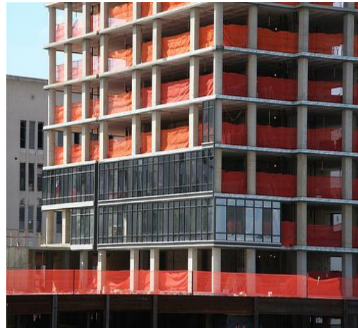
Fig. 2. Showing flat slab structure
