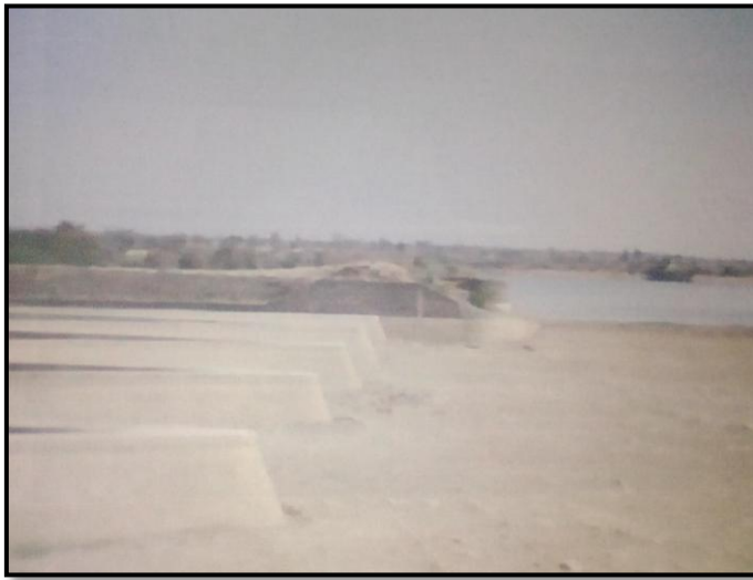
Fig. 14.Side View of Labyrinth Weir
