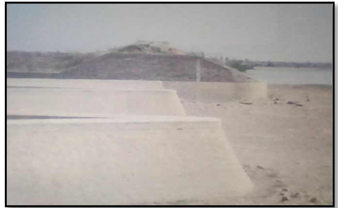
Fig. 11. Side View of Labyrinth Weir
