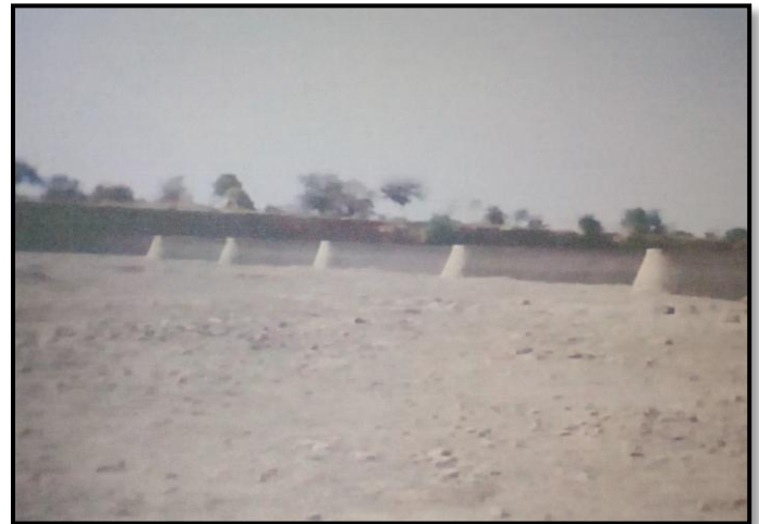
Fig. 12. Front View of Labyrinth Weir
